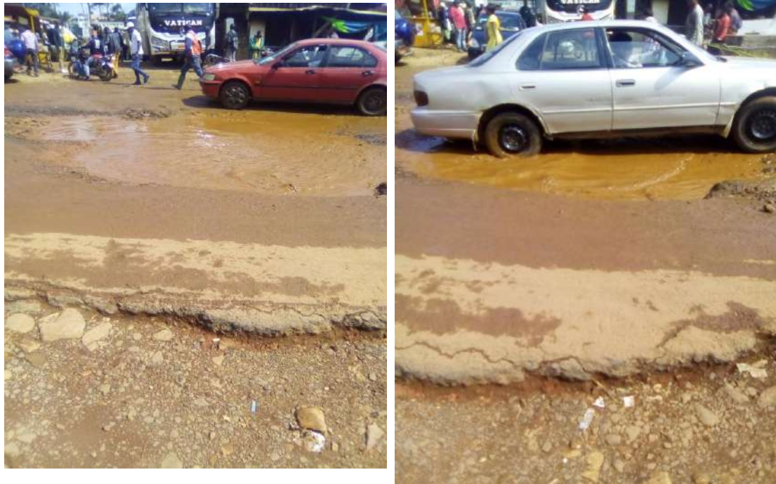
Photo A; Pothole at City Chemist Bamenda Photo B; Pothole at City Chemist Bamenda
