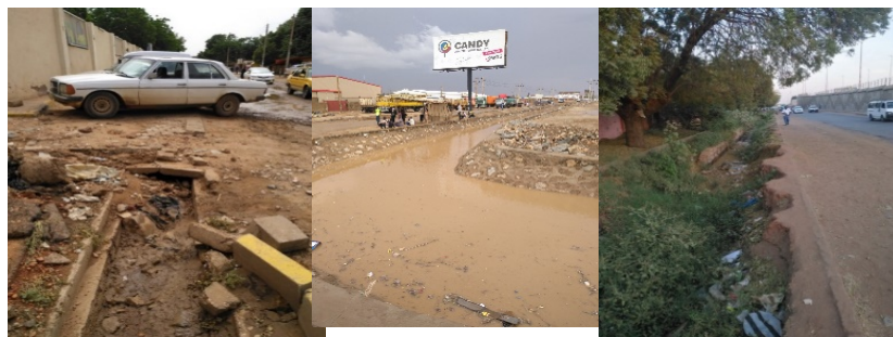
Fig. (4) Lack of maintenance and accumulation sediment and garbage, catching only direct rains with no outlet.
