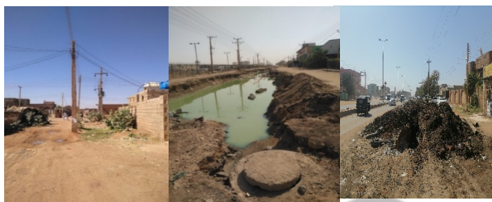
Fig. (3) Sewers, water mains left open for years after maintenance and random electrical poles.
