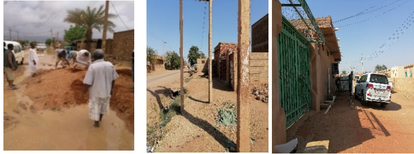
Fig. (6) Construction residue, backfilling soil and overreaching constrain storm movement
