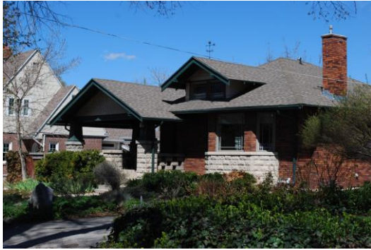
Figure 1. The architectural character of the building incorporates a variety of traditional design characteristics such as external porch, deep eaves, natural ventilation and solid masonry construction, ensuring efficient energy management and conservation.
