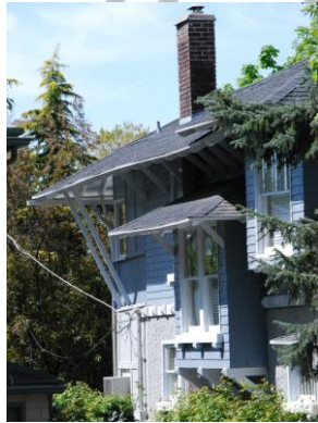
Figure 3. Projecting eaves provide protection from precipitation and solar exposure.
