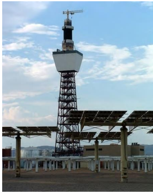
Figure 4-2: Tower and heliostats used in solar power plants 1 and 2
