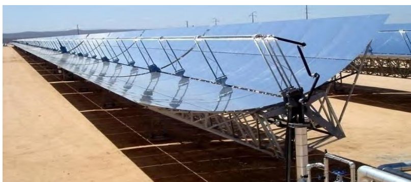
Figure 2: Linear shaped parabola power plant
