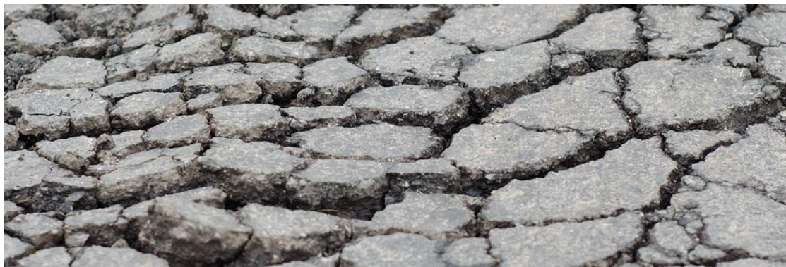
Figure 2 Recycled Asphalt Mix
