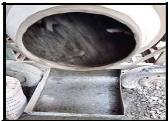
Figure 14: Final mixing of concrete
