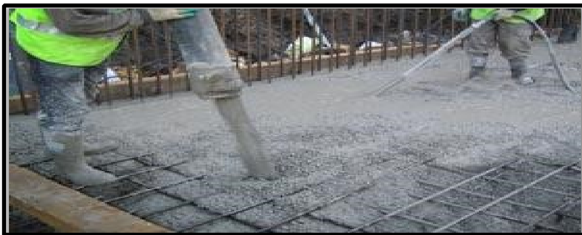
Fig 4: Showing that workability is more and pumping will be easy.
