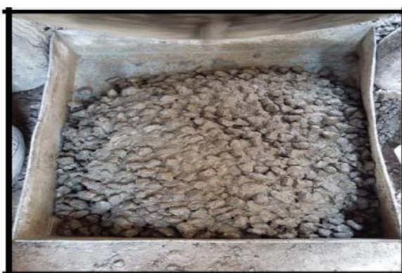
Figure 15: Discharging of concrete from mixer.
