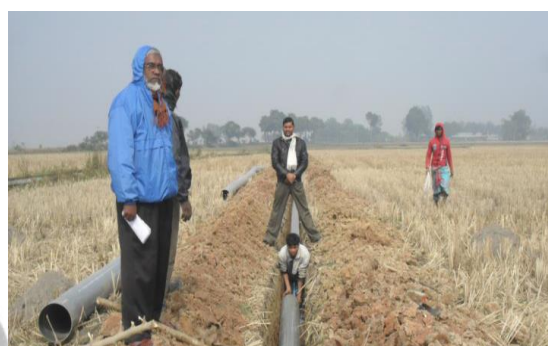
Laying of uPVC pipe in an Irrigation Scheme.
