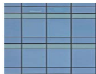
Figure 4.4 – Curtain wall (Source: F.A.S Lubis and P.W Dari)
