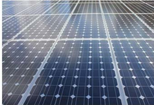
Figure 4.2 – Use of Solar Panels as An Additional Energy Producer (Source: F.A.S Lubis and P.W Dari)
