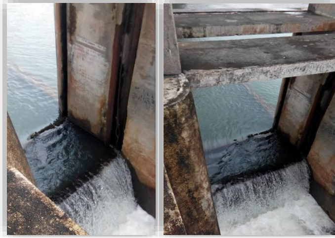
Figure 10 - NIA Existing Water Level Monitoring System
