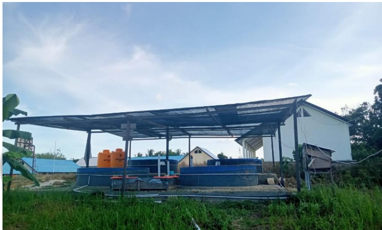
Figure 2. The condition after the biofloc tank has been built
