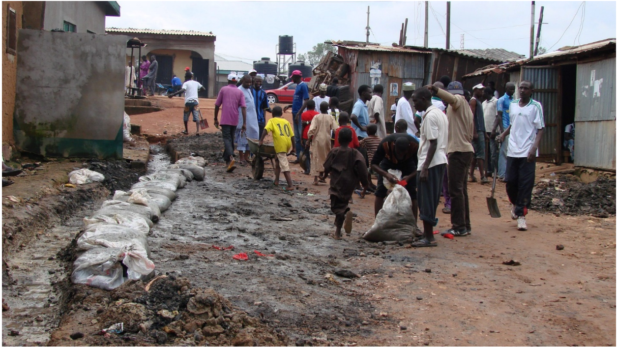
Plate 1: JUKDA Rehabilitating a Drainage
