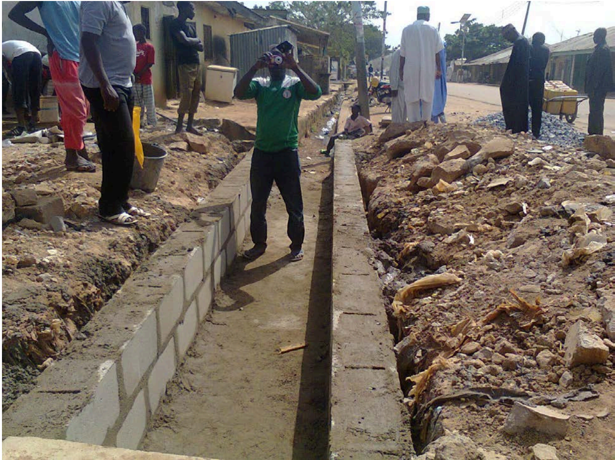
Plate 4: JUKDA constructing a Drainage
