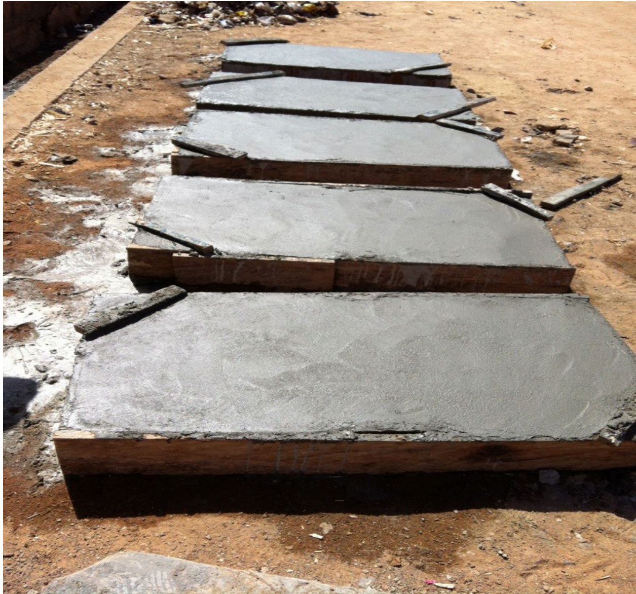
Plate 6: JUKDA's Slabs ready to be placed on a Drainage
