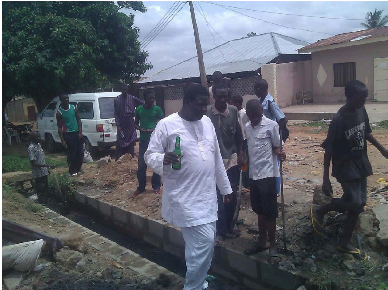
Plate 5: JUKDA Rehabilitating a Drainage
