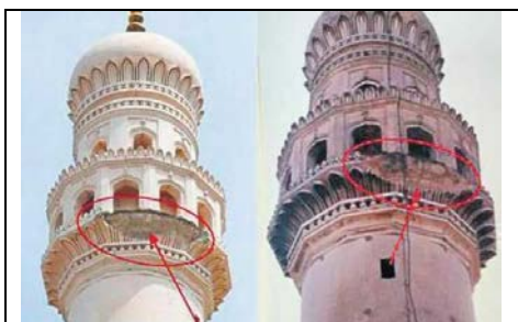
Fig No: 01 – Charminar cracks https://www.livemint.com/
