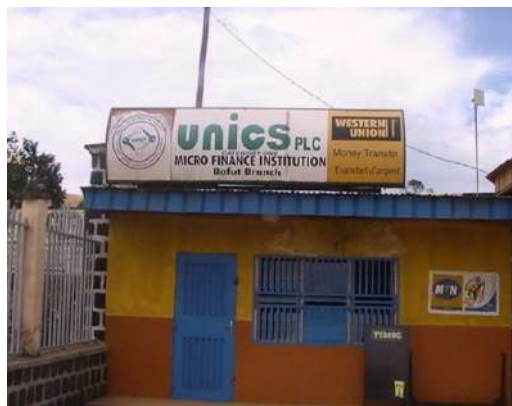
Photo 6: Unity Cooperative Credit Union, Njinteh-Bafut
