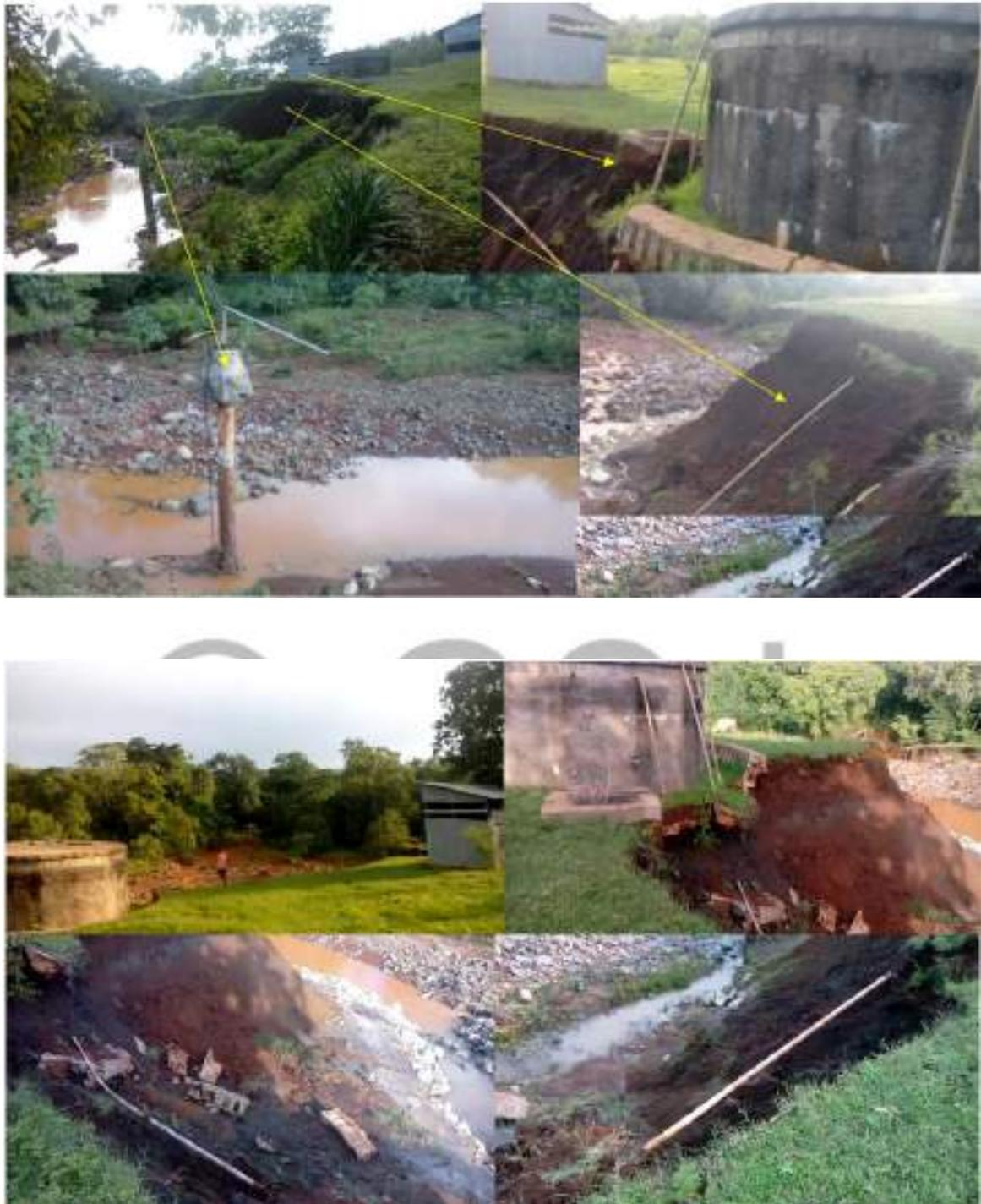
Figure 3:6 Deep well source of water supply of Bullen Town (demolished due to riverbank erosion)
