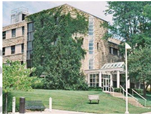
Fig 6: Rockhurst University, Kansas City, Missouri, makes good use of climbers and trees to limit heat penetration into the structure. (Ogunsote,Prucnal-Ogunsote,Adegbie, 2005)
