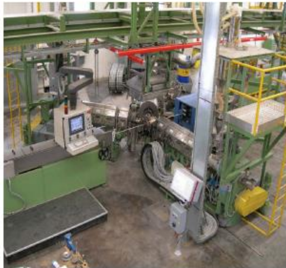
Fig. 8 No vulcanization line: cooling system device is installed after triple extrusion.
