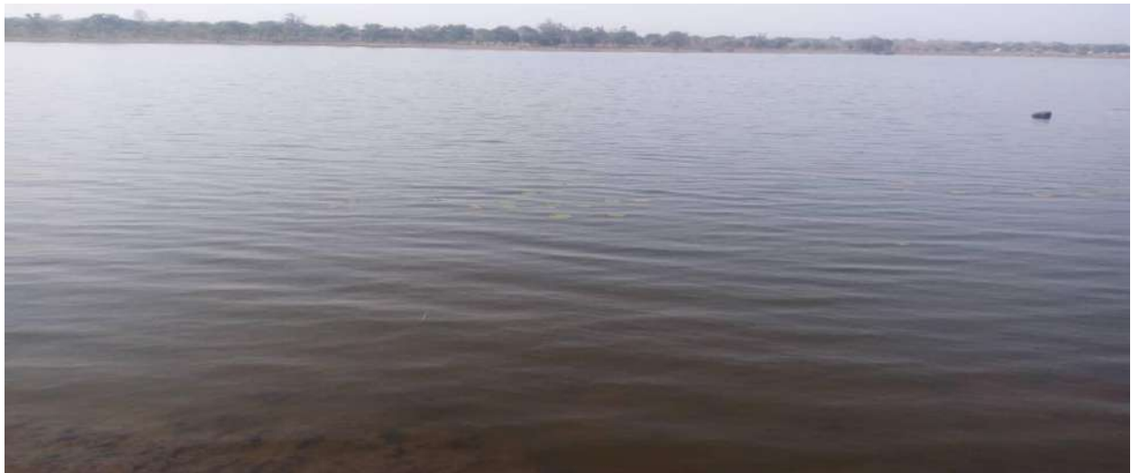
Figure 1: Irrigation dam at Sankana
