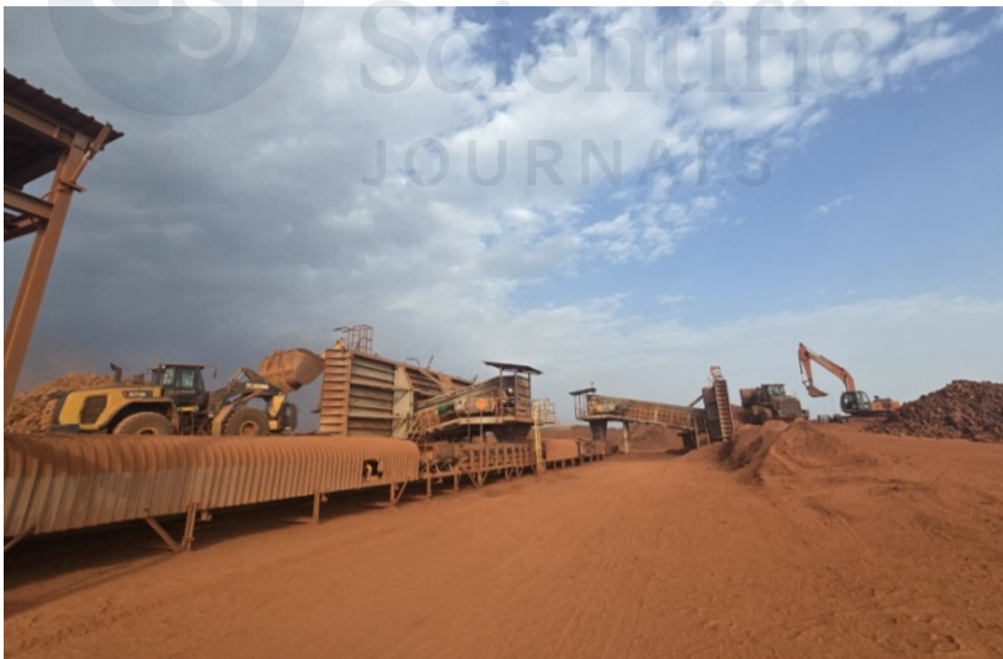
Figure 3: Front end loader feeding dozer trap (Source:[10])
