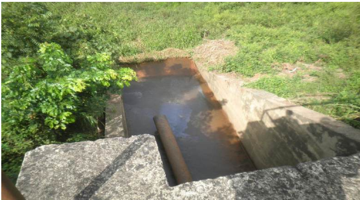
Plate 73: showing irrigation system attached to the failed earth dam.
