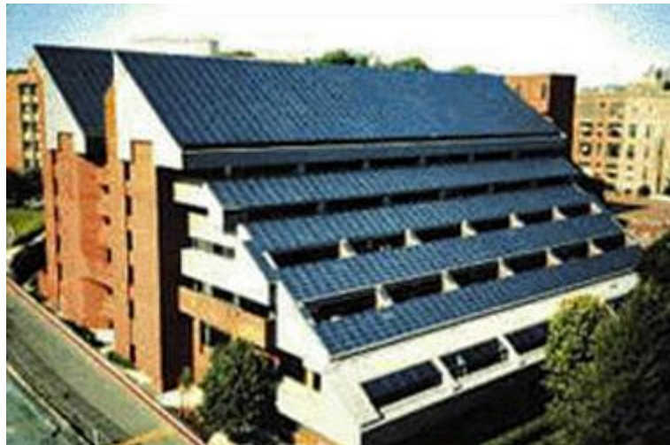
Figure 9. Building Integrated Photovoltaic Panels [BIPV]
