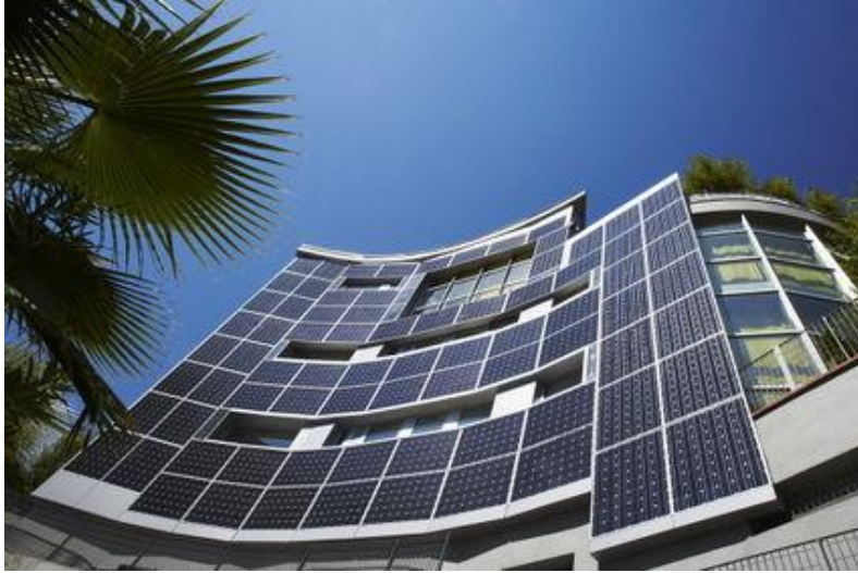
Figure10 Building Integrated Photovoltaic Panels [BIPV]
