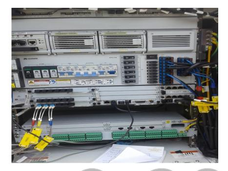
Fig 1.0: A typical Baseband unit for Base Transceiver Station
